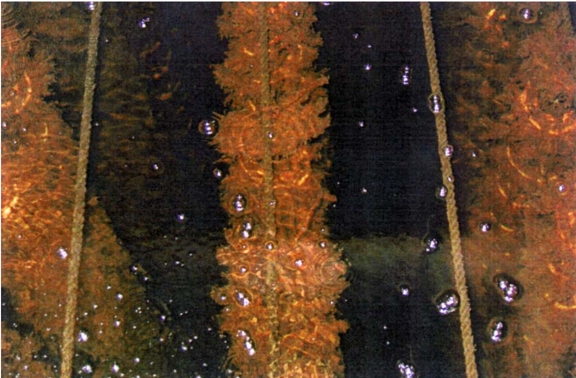
Treated effluent in clarification chamber, liquid has become clear with low turbidity
